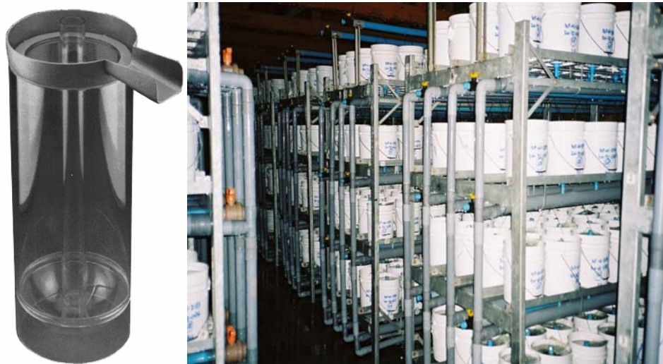
Figure 3. Egg incubators - detail of silo or zoug jar incubator and commercial silo incubator system
